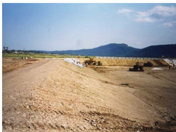
Figure: EU funded Engineered Landfill, Romania
